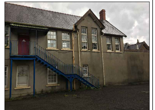
EXISTING REAR VIEW
